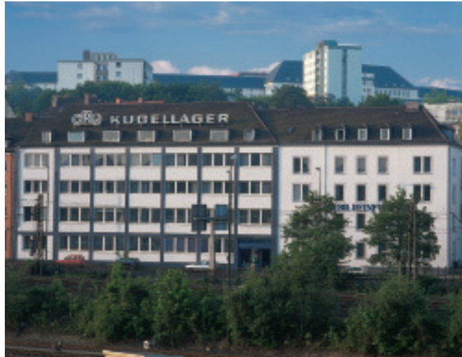
Administration and production facilities in Würzburg
